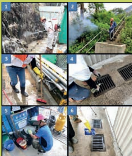
Anti-mosquito Breeding Control System 防止蚊卵繁殖及控制系統
