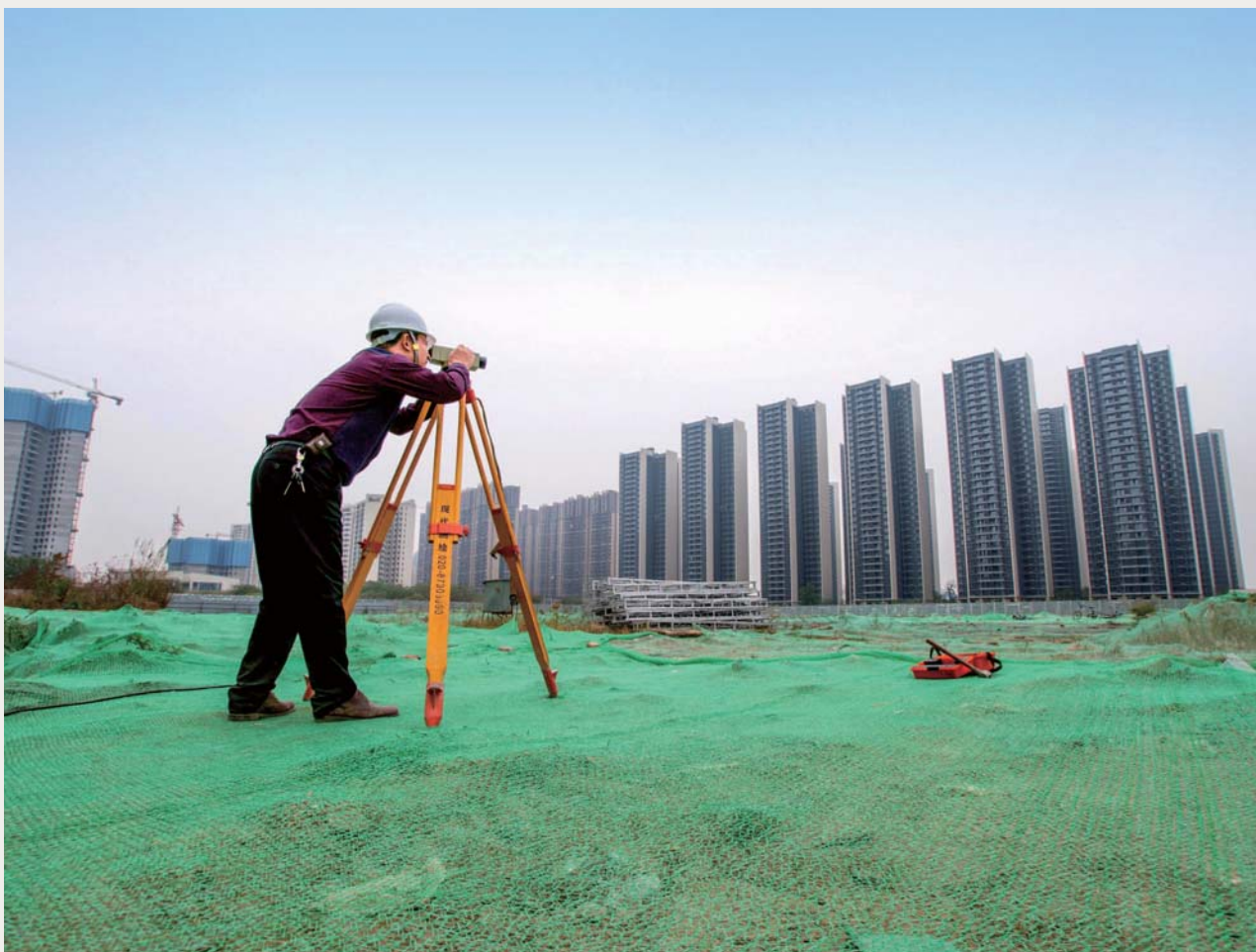
The new residential project under survey in Sanshui, Foshan 佛山三水新住宅項目進行測量工程
