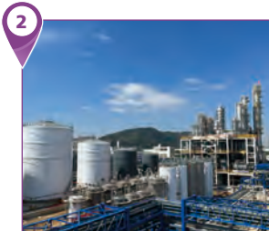
位於廣東珠海的溶劑廠房 The solvents plant in Zhuhai, Guangdong
