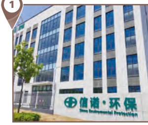
位於山東青島的化學氣體治理設備廠房 The chemical vapour treatment equipment plant in Qingdao, Shandong
