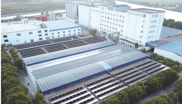
The solar PV modules installed in the flour plant in Jintan 於金壇麵粉廠所安裝的太陽光伏組件
