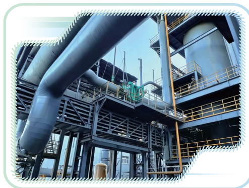
Equipment for blast furnace taking-off blast gas recycling 高爐休風放散回收設備
