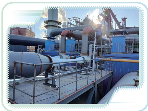
Equipment for blast furnace taking-off blast gas recycling 高爐休風放散回收設備
