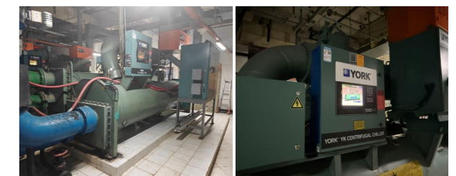
Before and after chiller unit retrofits
