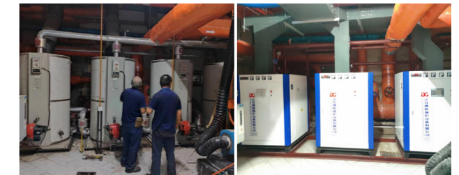
Before and after boiler retrofits
