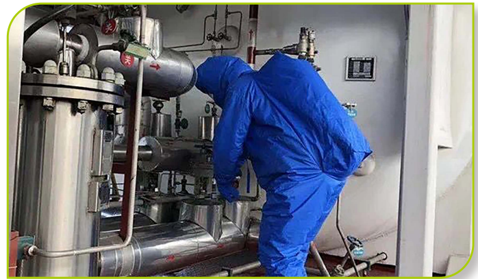
Gas leakage emergency drill 燃氣洩漏應急演練
