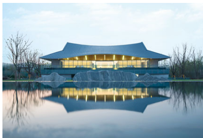
蘇州吳中區西山項目 Suzhou Wuzhong District West Mountain Project
