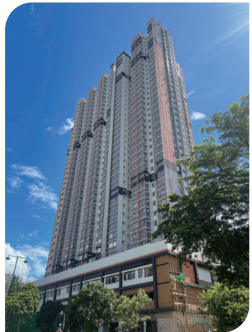
Public housing development at Hin Fat Lane, Tuen Mun 屯門顯發里之公共房屋發展項目
