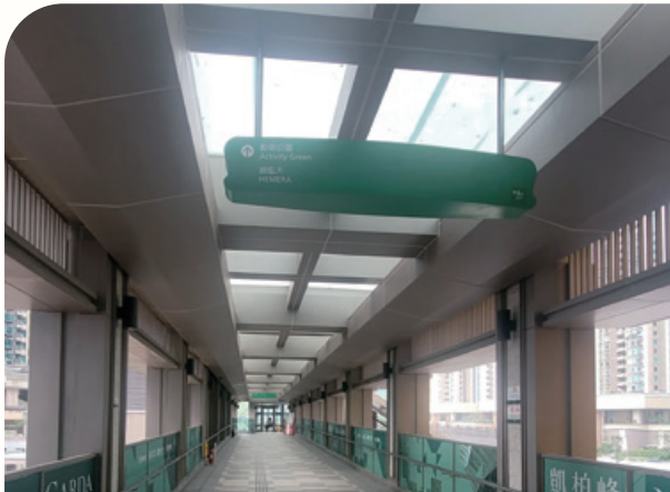
Proposed residential development at TKOTL 70RP, Phase 11, Lohas Park, Tseung Kwan O – Supply and installation of baffle ceiling and gypsum board ceiling system 將軍澳日出康城第11期將軍澳市地段第70號之餘段之建議住宅發展項目－供應及安裝條子天花及石膏板天花系統
