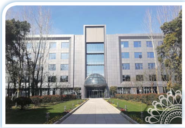
Windows and glass curtain walls are made of insulating broken bridge glass which can help reducing energy loss.
