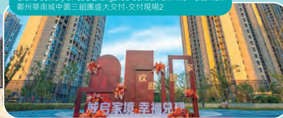
Grand delivery of CSC Zhengzhou Central Park Trio – Site view 鄭州華南城中園三組團盛大交付-交付現場2
