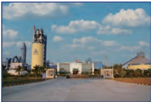
Dugongo Cement, Mozambique
