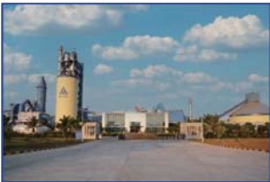
Dugongo Cement, Mozambique
