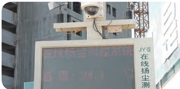
Dust and noise monitoring system 揚塵雜訊監測系統
