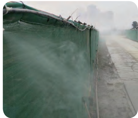
Chengdu Cadiere project-fence and spray 成都卡地亞項目 — 圍擋噴淋
