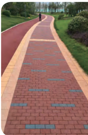
Permeable pavement 透水鋪裝
