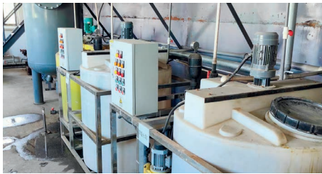
氣浮機改造 Steam floatation machine upgrading
