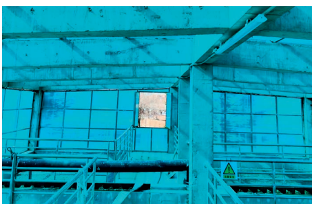
水解酸化池 Hydrolytic acidification pool works
